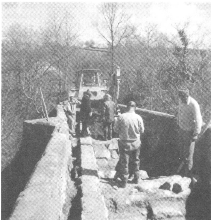
'Digging out' Wenford Bridge in April 1977
