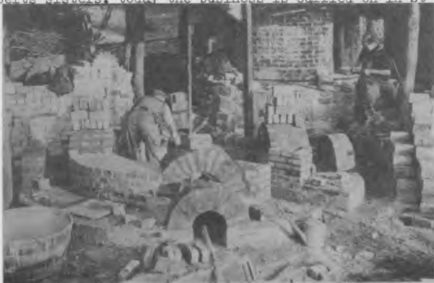
Building the Wenford Bridge kiln, 1949
